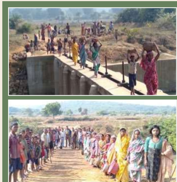
Villagers are carrying stones to the other end of the bridge
